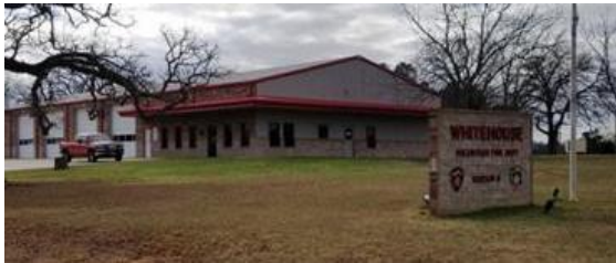
Figure 134: Whitehouse VFD, Station 1
